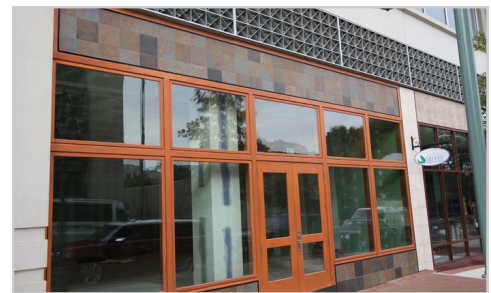
Above: Transoms and mullions add detailing and limit the amount of glass to be replaced if broken.
