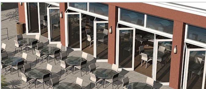
Above: Bi-folding doors can create a more open connection between inside and outside and allow for social activities to spill out onto the street.
